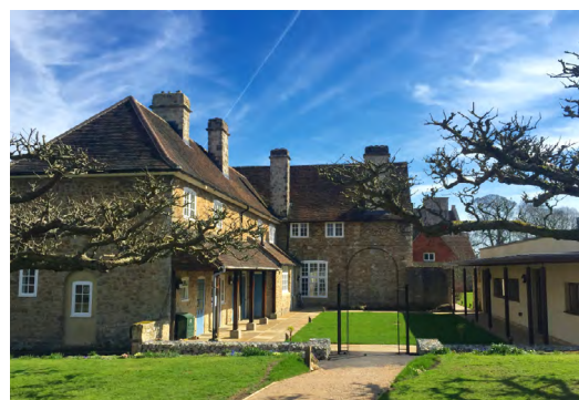
ST BENEDICT'S CENTRE, WEST MALLING
